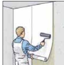
4. Firmly press down the lengths of wallpaper with a foam rubber roller.
