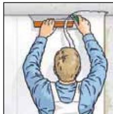
6. Cut off excess wallpaper in the corners with a wall-papering palette knife and a Stanley knife or using scissors.
